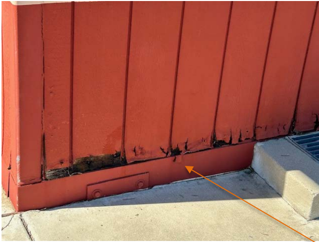
Example of T-11 repairs/replacement
