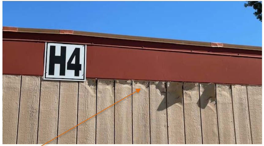
Example of T-11 repairs/replacement
